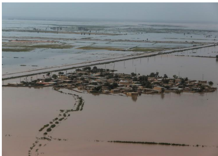
Figure 8: An aerial view of flooding in Khuzestan province, Iran, April 5, 2019
