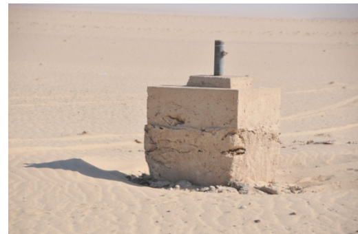
Figure 2.2: Boundaries markers were damaged due to the test of time
