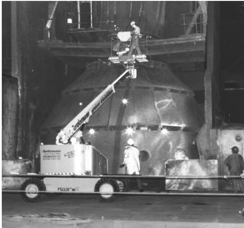
Fig. 6: Signalling the converter by the assistance of a lifting jack
